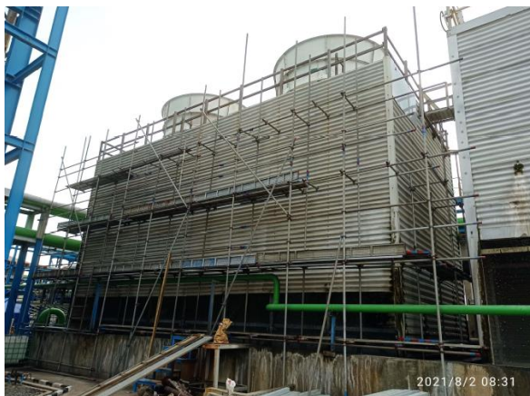
Figure 3. When installing scaffolding on a cooling tower
