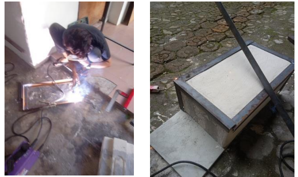
Figure 12. Welding process and manufacture of furnace frames
