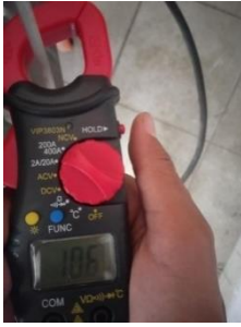
Figure 15. The process of measuring amperes using an ammeter
