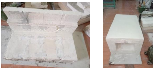
Figure 11. The process of uniting all refractory bricks
